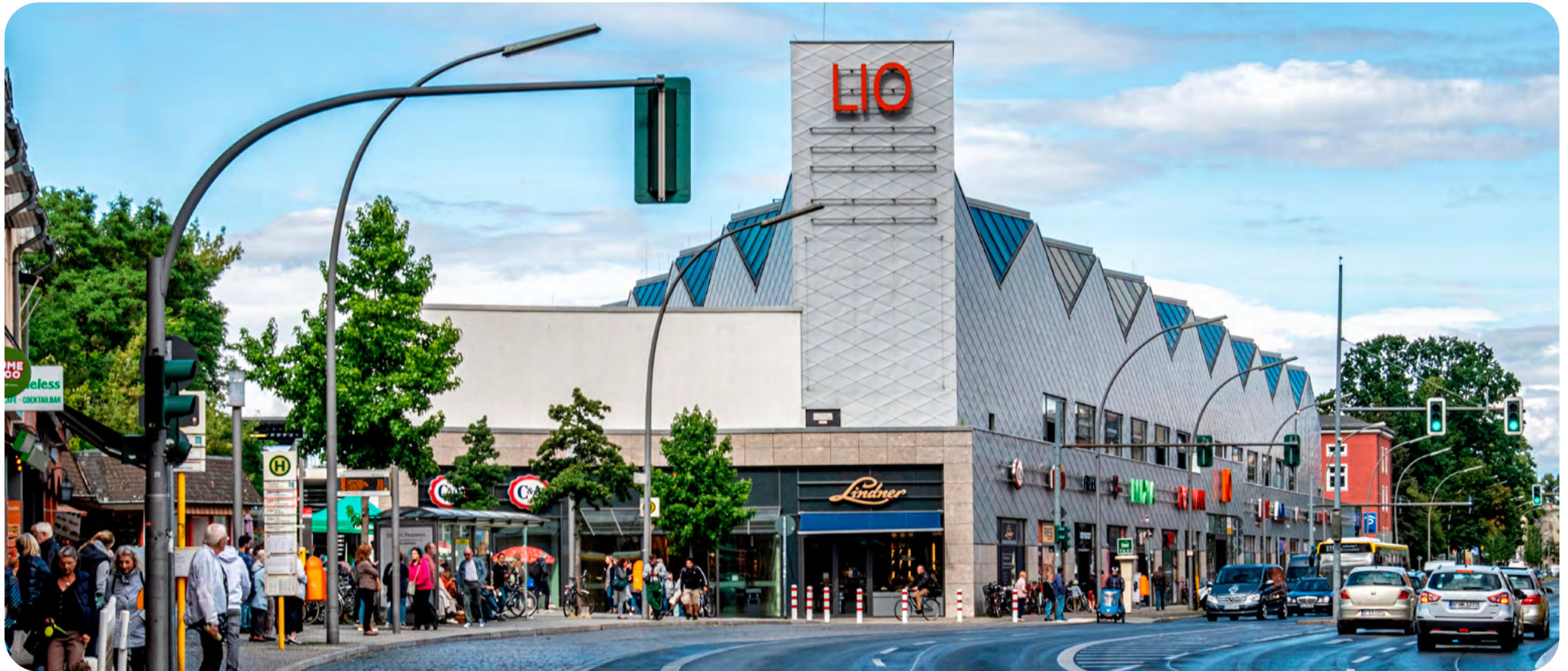
The car park at the Lio shopping mall (Berlin), with 308 parking spaces, expands Saba's presence in Germany.
